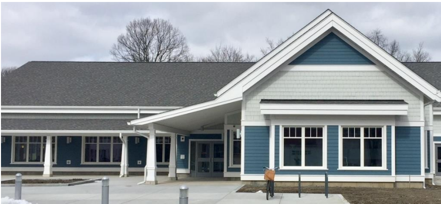
Top: present day building
