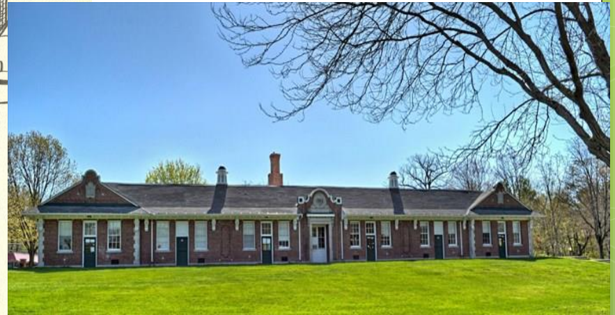
↑ Present day building
